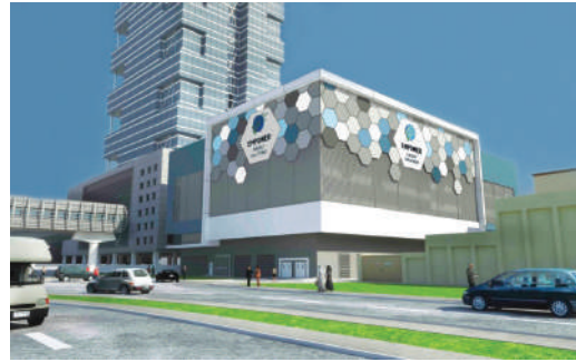
▲ TECOM District Cooling Plant, Dubai, UAE
