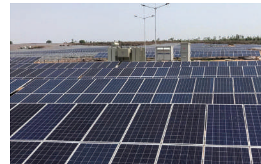
▲ 750 MW Solar Power Project in Rewa, Madhya Pradesh
