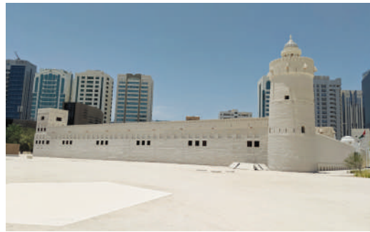
▲ Qasr Al Hosn at Abu Dhabi, UAE
