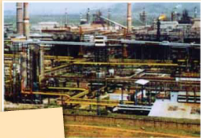
Electrical power distribution system for coal handling unit.
