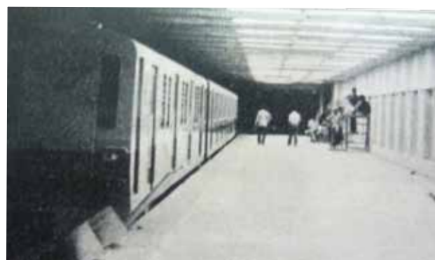
Underground air conditioning & ventilation for India's first Metro Rail in Kolkata – three stations including Park Street, the longest.
