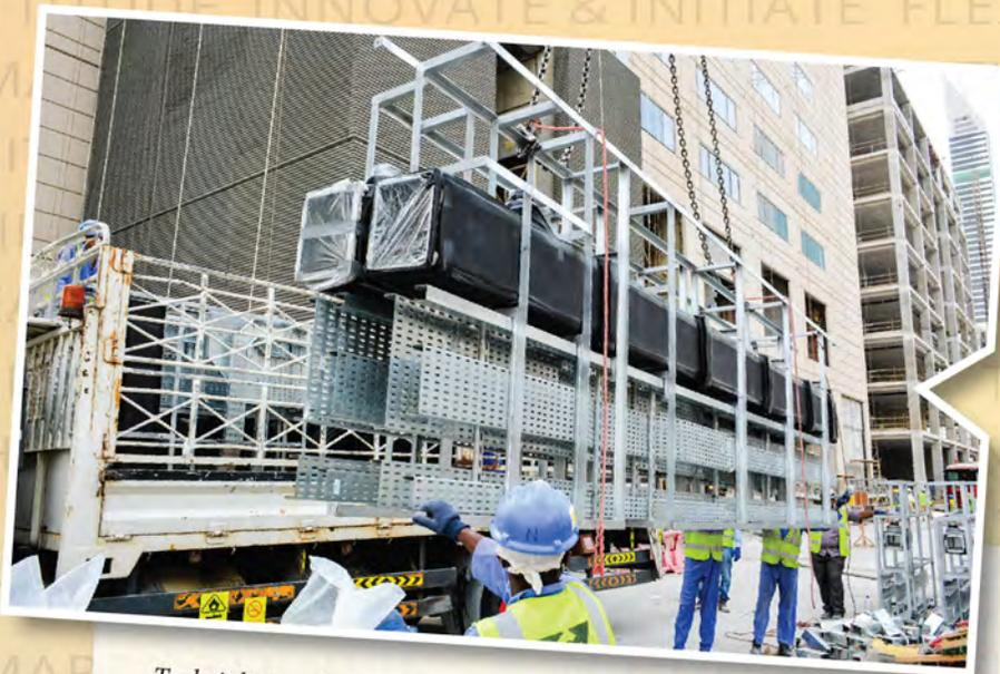
*To do it better, do it in advance. That's the new motto at Voltas' International Operations. Pre-fabricated modules are manufactured off-site and later assembled and installed on-site. The payoff – on time delivery, less wastage, better manpower utilization, and a safer work environment.*
