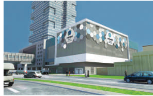
▲ TECOM District Cooling Plant, Dubai, UAE
