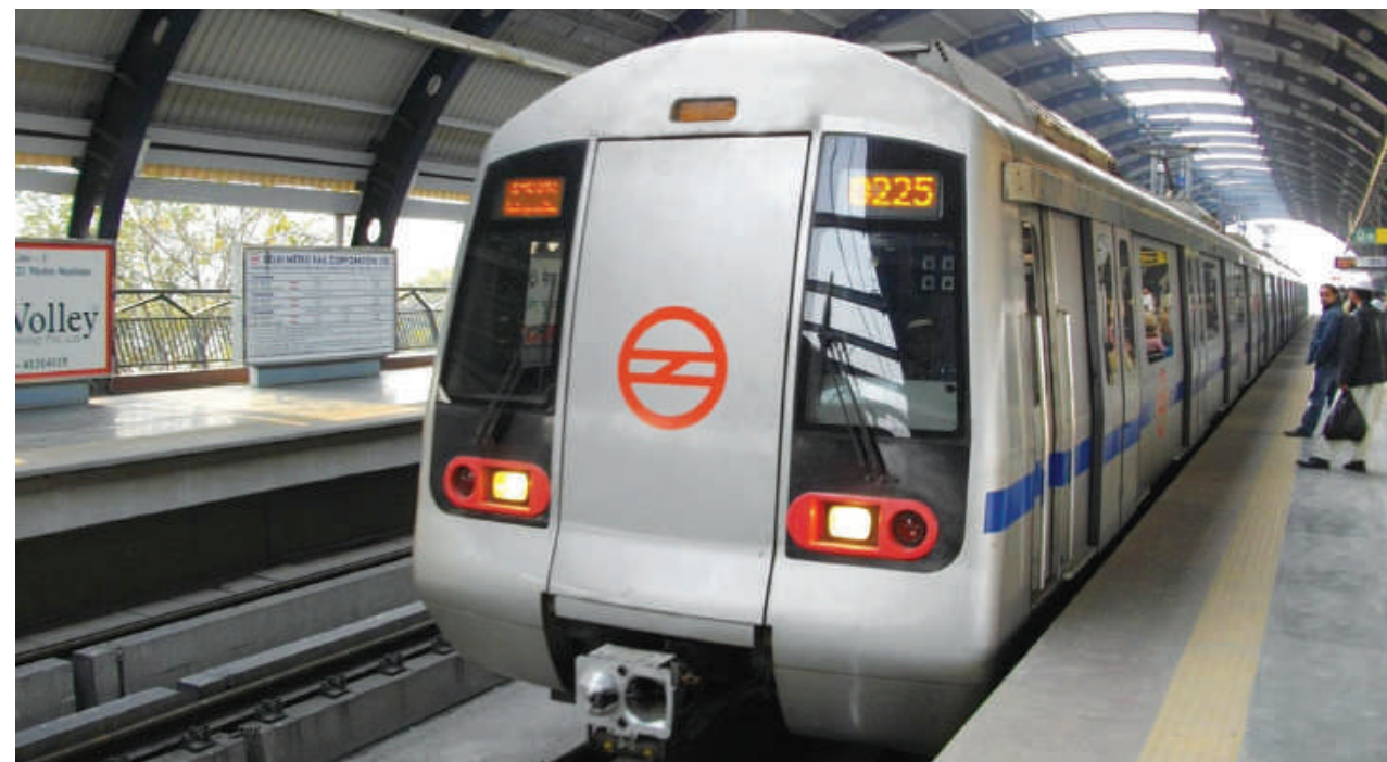
▲ Delhi Metro Rail Corporation Project
