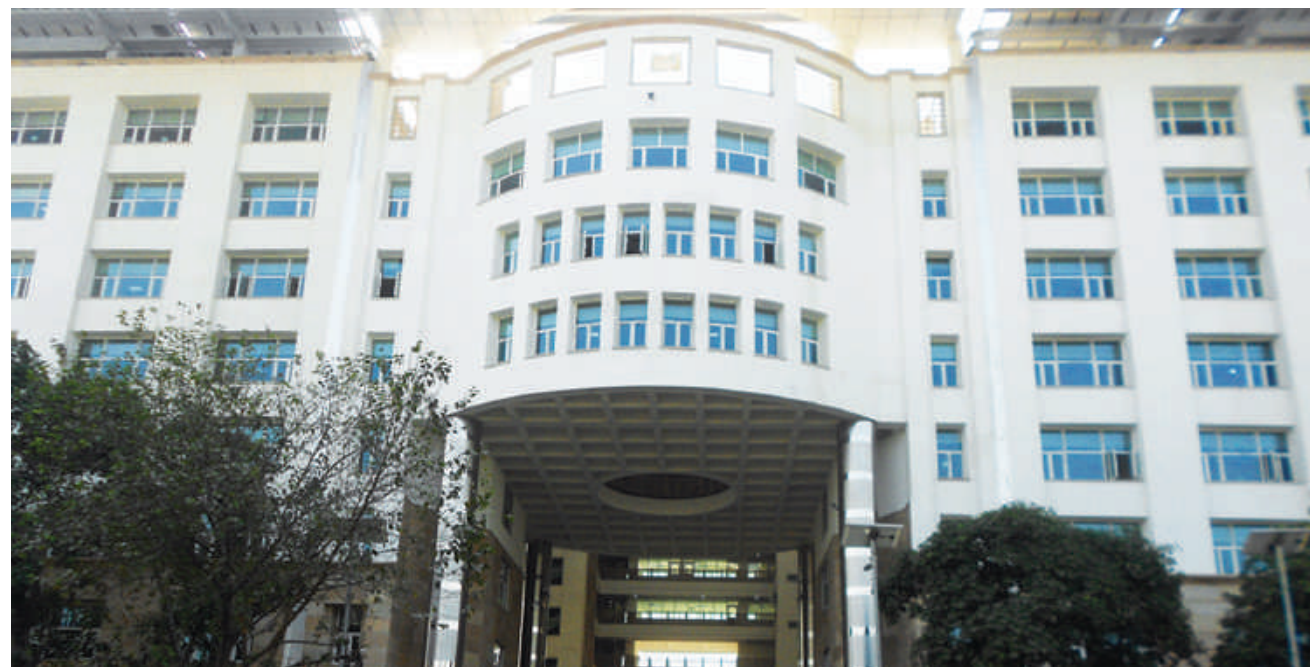
▲ Indira Paryavaran Bhawan - India's first net zero energy green building, New Delhi
