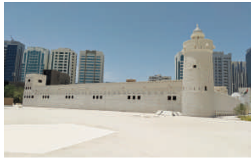
▲ Qasr Al Hosn at Abu Dhabi, UAE
