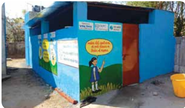
Waghodiya Kanya school urinal after intervention
