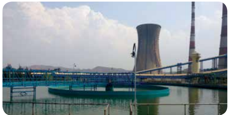
Water Treatment and Management Project for Karnataka Power Corporation Limited
