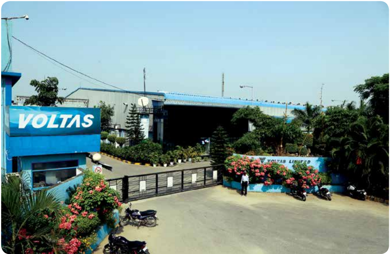
Voltas Pantnagar Facility
