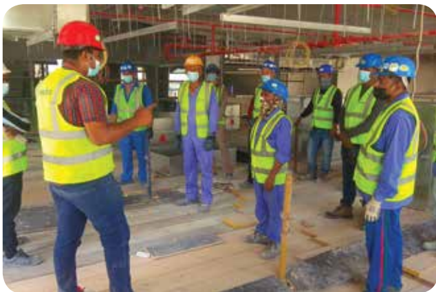
Project site - Safe usage of Hand & Power Tools
