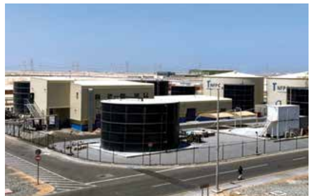
|||||| National Food Products Company - Effluent Treatment Plant, Kizad, Abu Dhabi, UAE
