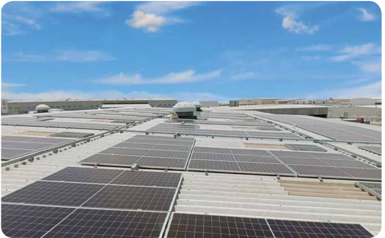
Voltas commissions first solar project in Dubai For SirajPower
