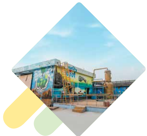
Bihar Urban Infrastructure Development Corporation, Beur
