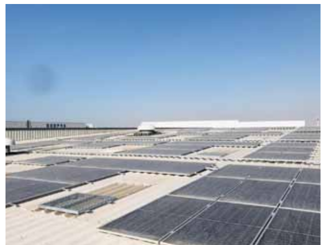
On site images of first Solar Project in Dubai
