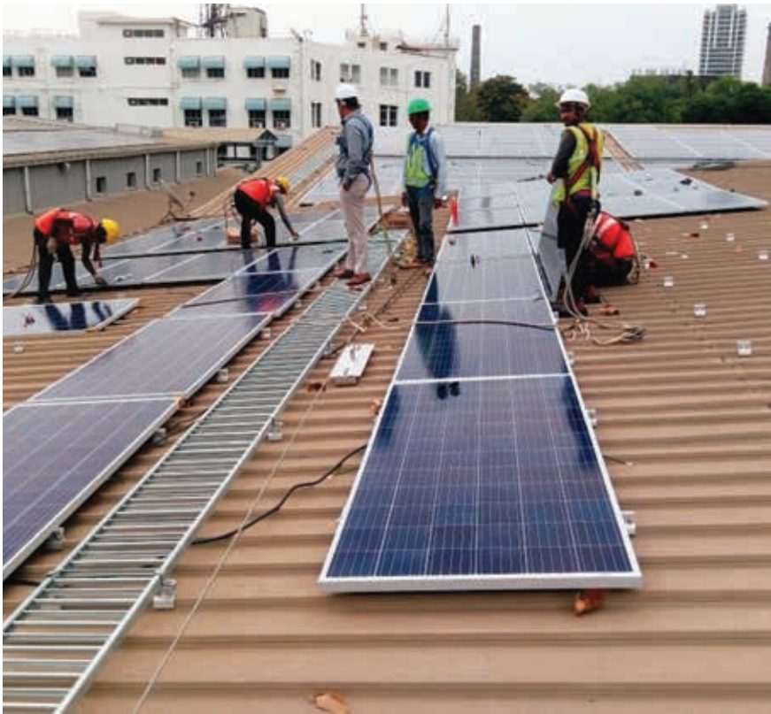
▲ Installation of 1563 solar panels in Voltas HQ at Chinchpokli, Mumbai
