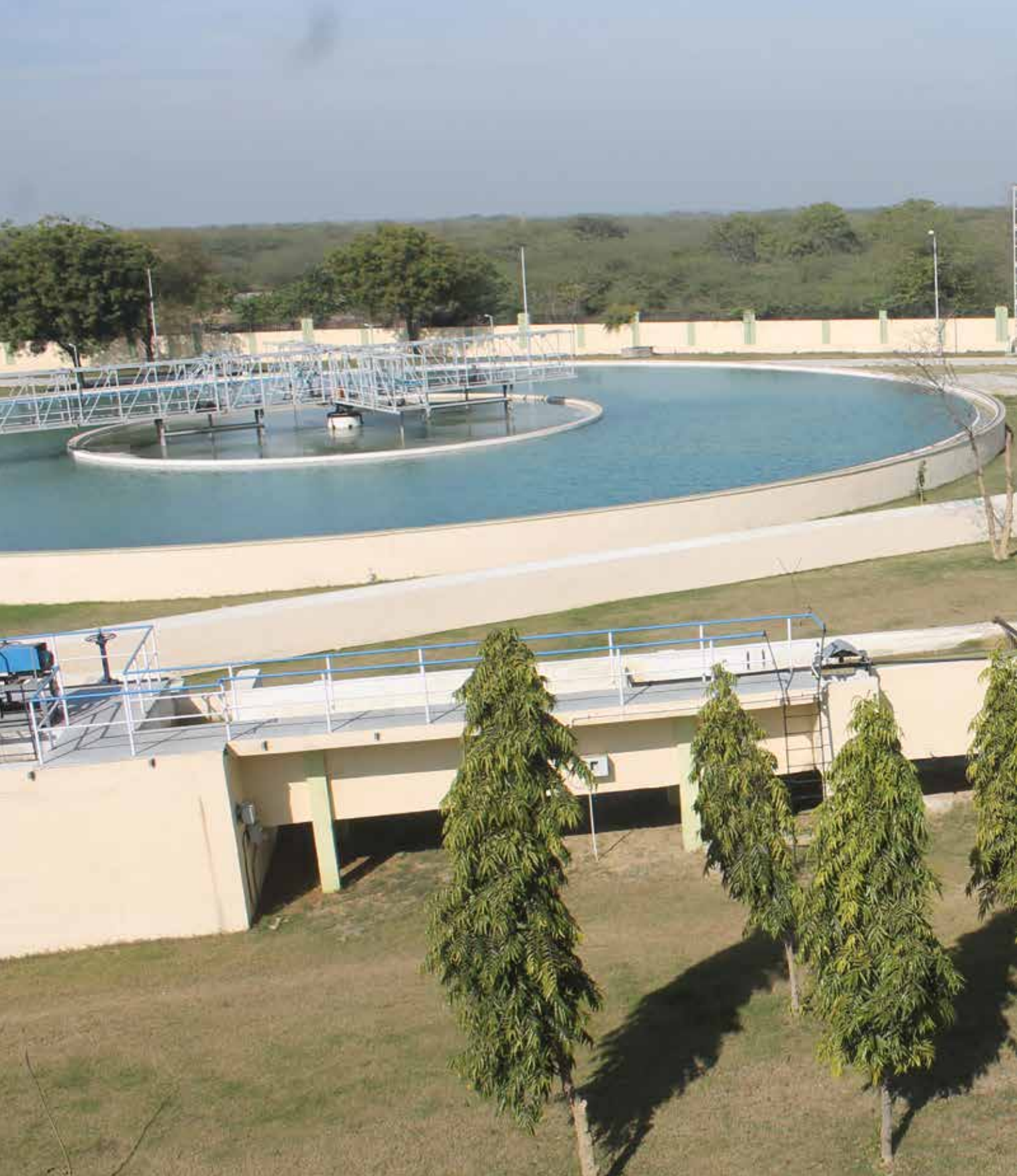
▲ Water management and treatment project at Uttar Pradesh Jal Nigam (UPJN) site
