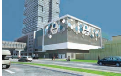
▲ TECOM District Cooling Plant, Dubai, UAE
